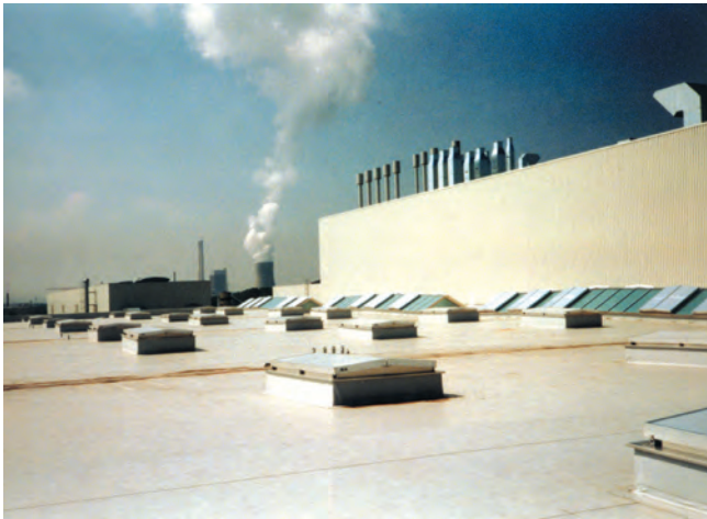
PHOENIX PX2 on upstand and in glazing
